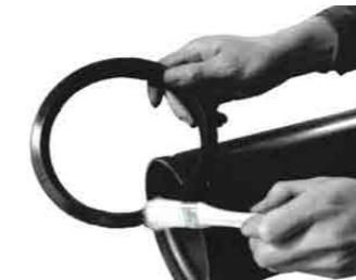
2. Lubricate gasket
