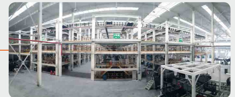
Threading, Air Pressure Test, and Anti-rust Treatment
